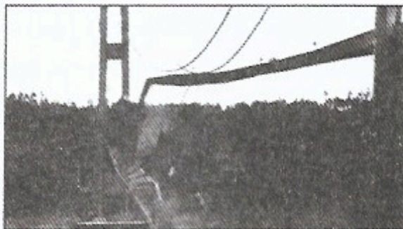
Bridge collapse Jambatan runtuh
