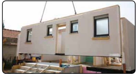
Prefabricated houses are built in a shorter time and with a lower construction cost.
