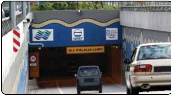
The Stormwater Management and Road Tunnel (SMART) can reduce loss and traffic accidents caused by flash floods in the city.
